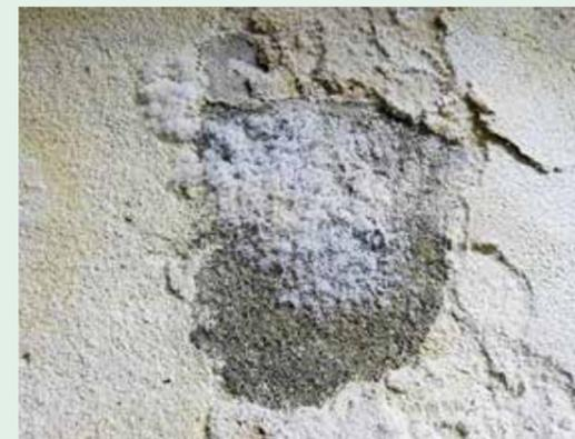
If water penetrates the masonry, salts are often brought to the surface. These salts recrystallise and cause “efflorescence”. The result is unsightly, usually white or yellowish stains on wallpaper or render. Efflorescence and crystallisation cause spalling.
