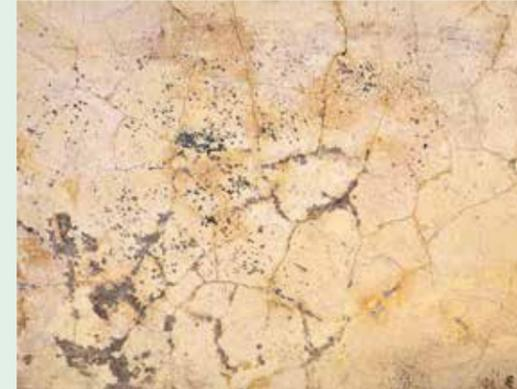
After the water has been pumped out, if cracks and/or spalling are visible on load-bearing and non-load-bearing structural components, then a structural engineer should assess the damage. If only the render has been damaged but the structure is still sound, in many cases the wall can be plastered over with suitable render material.
