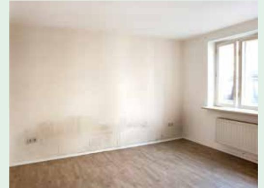
Visible mould after water damage is often only the tip of the iceberg. Microbiological analysis is therefore advisable prior to restoration. This provides the basis for developing and implementing a suitable mould remediation concept. Experts generally advise against using fungicides indoors.
