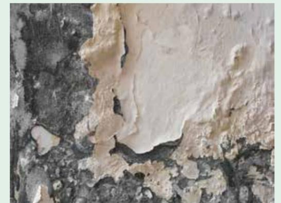
Increased moisture values in the masonry of building components in contact with the ground can result in various types of damage: efflorescence, flaking of paintwork and render, sanding of render and structural destruction of masonry or also corrosion damage to integrating steel beams.
